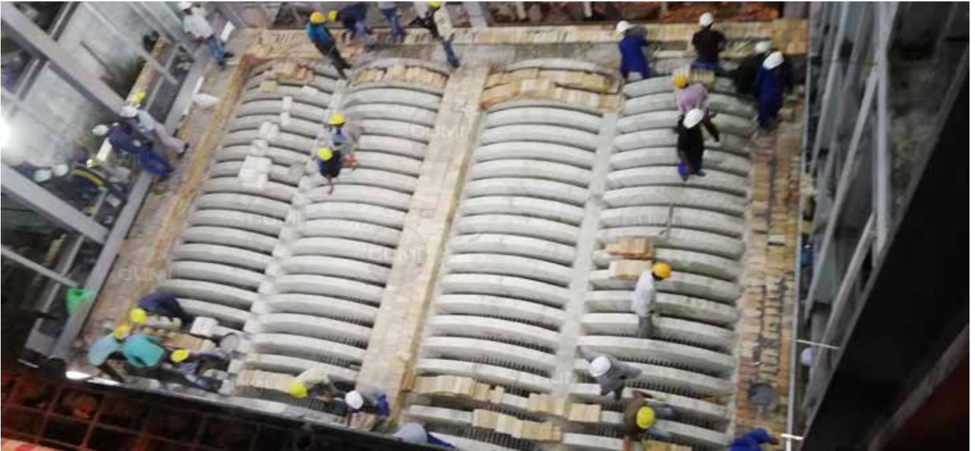
Rider Arch Construction at site
